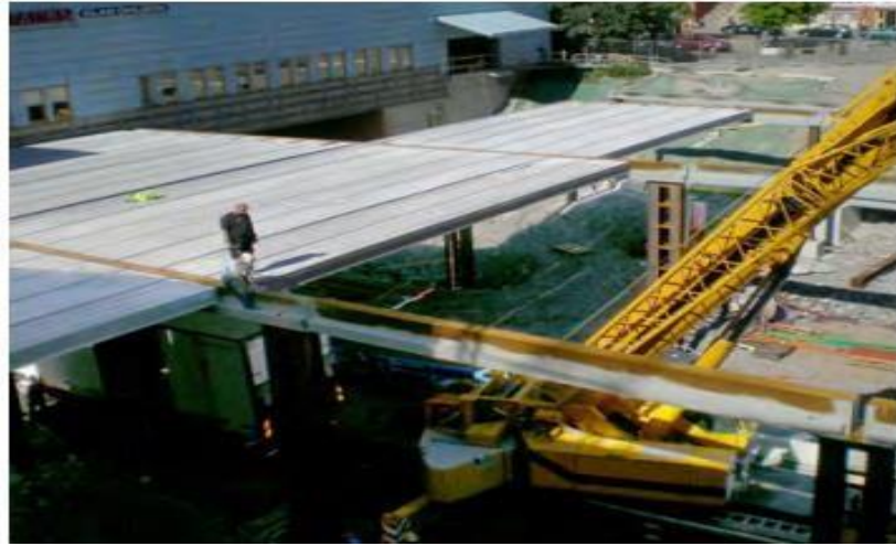
Figure 2.3: Construction of a Commercial Hub with a Half-Hour View
