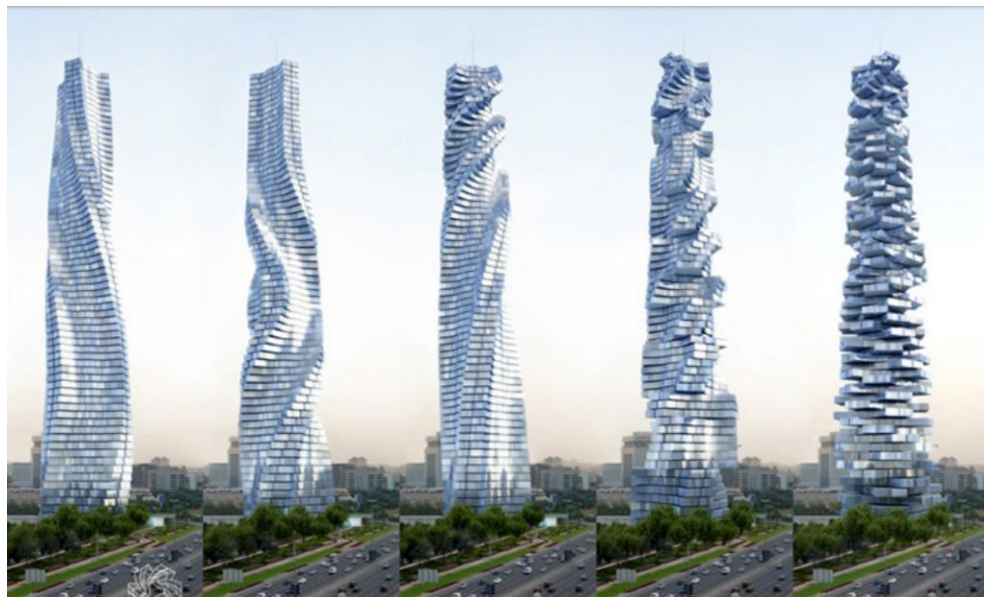
Figure 2.17: Dynamic Tower, Dubai, UAE
