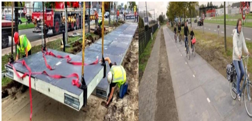
Figure 2.27: Pre-Fabricated Slabs of the Solar Panel
