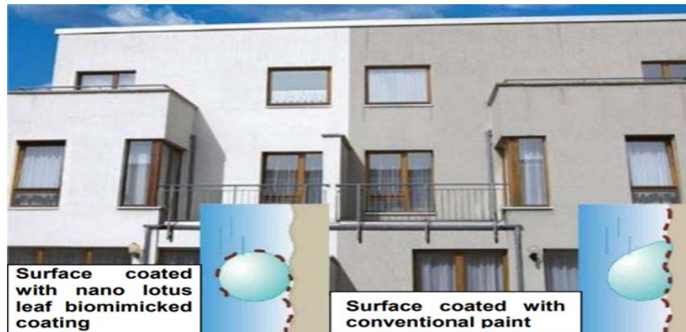
Figure 2.14: Comparison of Conventional and Nano Lotus Leaf Bio Mimicked Coating
