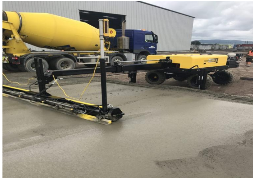
Figure 3.3: The Laser Controlled Concrete Finishing System.
